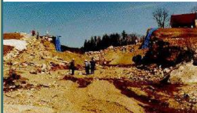
Alton dam breach, 1996
