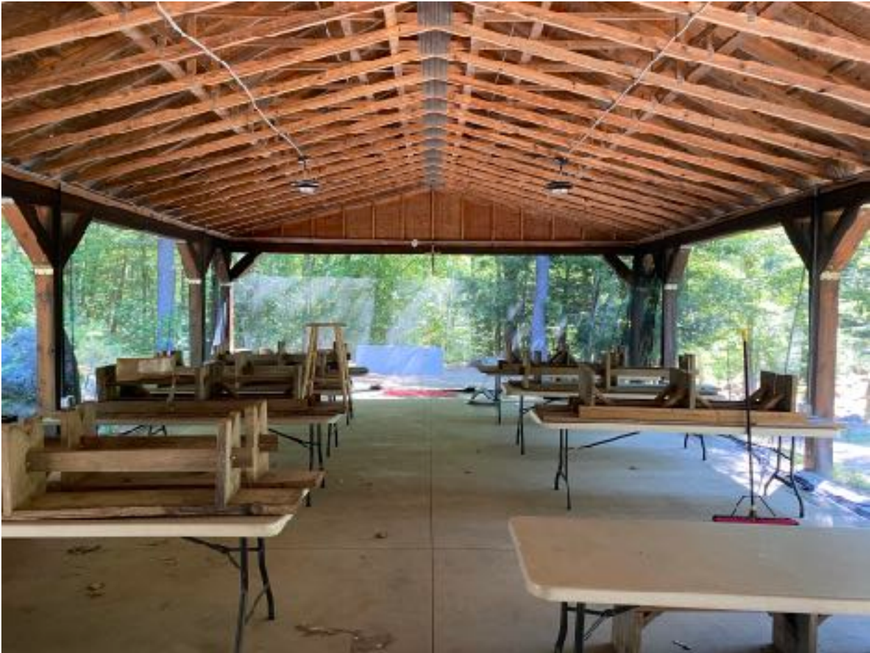
Fig. 16 - Dining Area Overview
