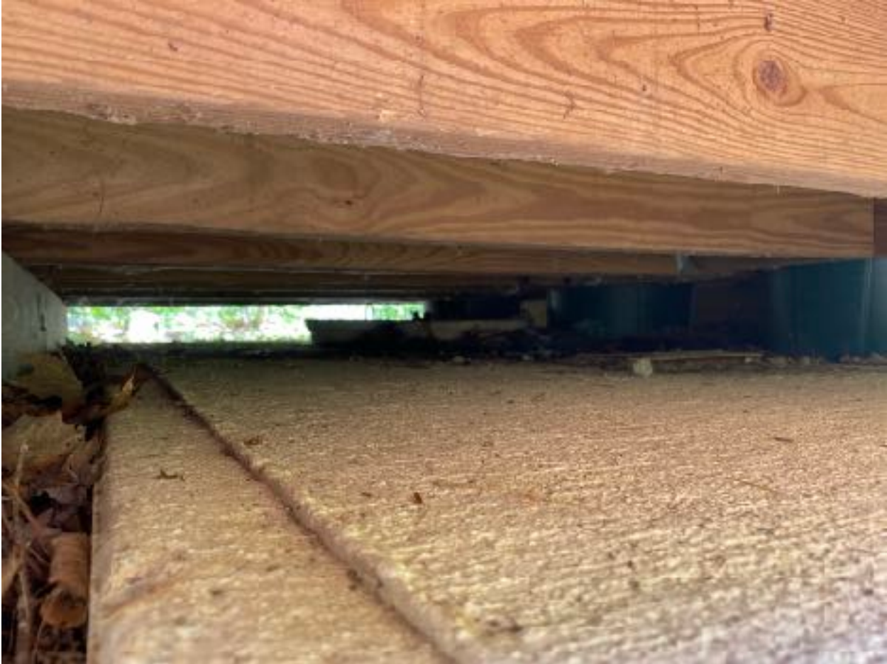
Fig. 20 - Main Area Outhouse Vault
