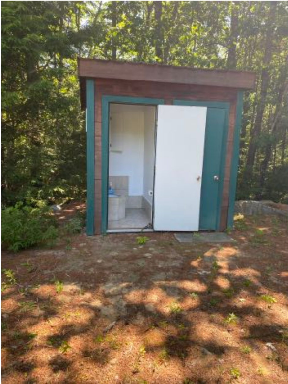
Fig. 24 - Southeast Field Area Outhouse
