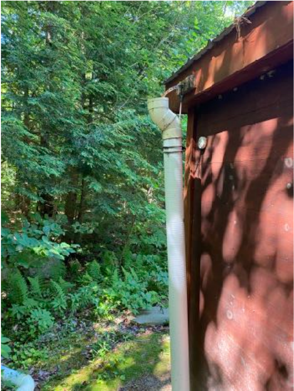
Fig. 23 - Southwest Field Area Outhouse Vent Pipe
