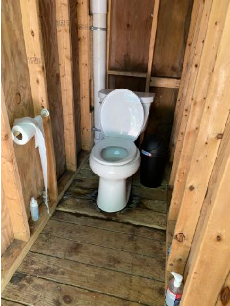
Fig. 19 - Main Area Outhouse Flush Toilet
