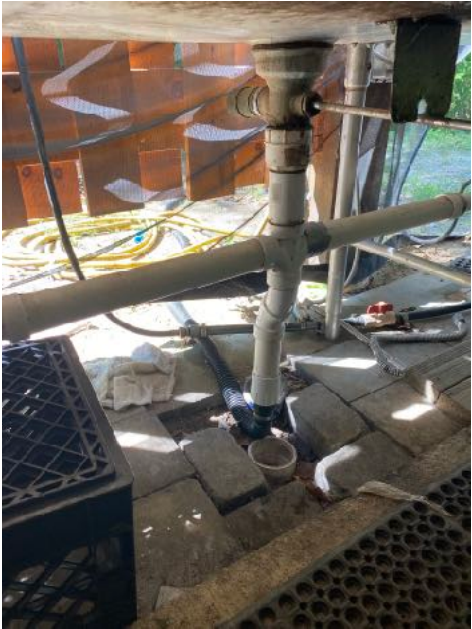
Fig. 8 - Kitchen Sink Plumbing
