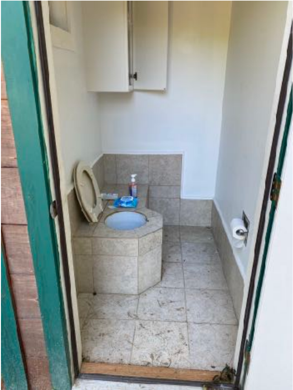
Fig. 25 - Southeast Field Area Outhouse Interior
