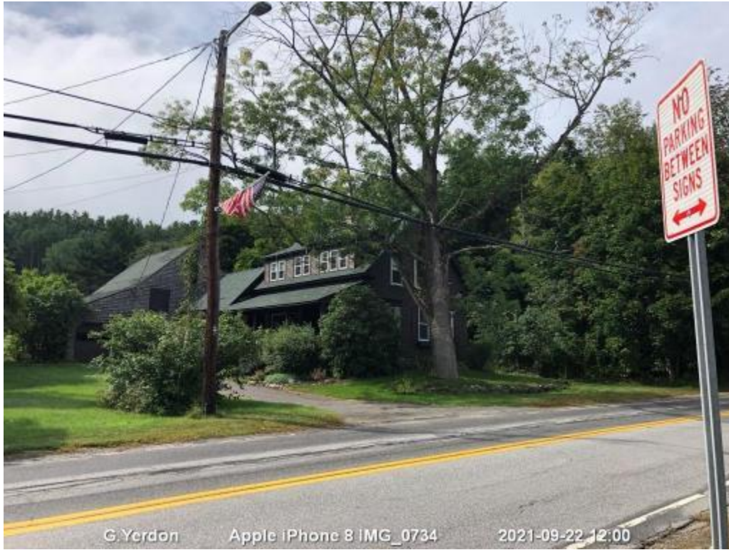
SCENE: View of 67 Plymouth Street. Photograph taken facing east.
