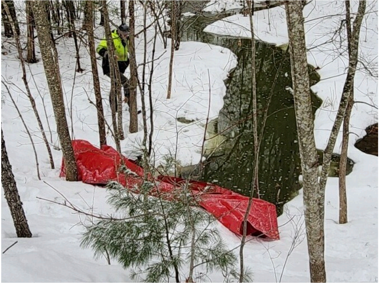
Fig. 5 - Green, cloudy fluid moving toward culvert under the driveway of 183 Whittier Highway. Culvert has been diked with red salvage cover - 01/16/2024
