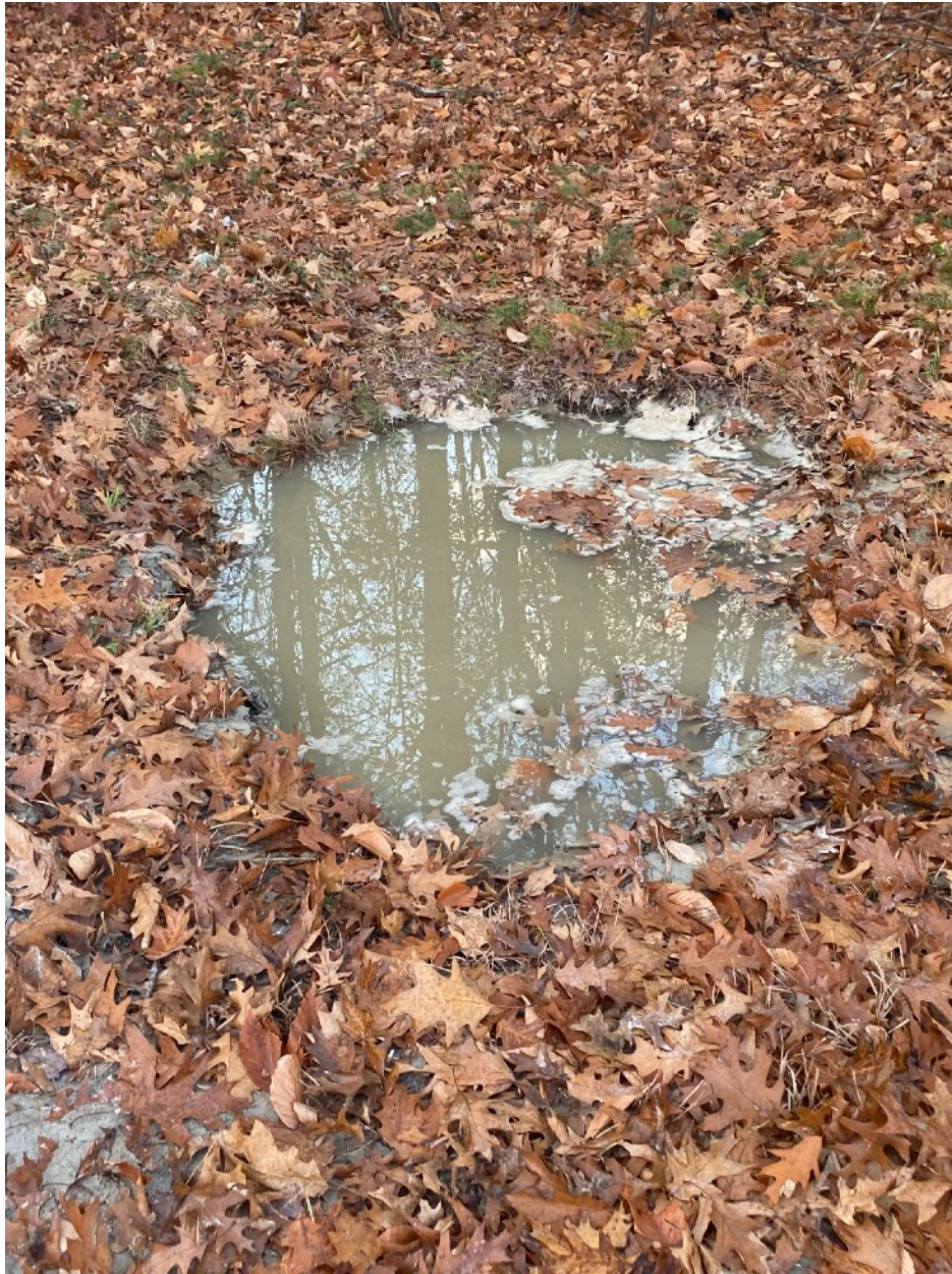
Fig. 2 - Clay-colored fluid collecting in and flowing out of an approximately 3 foot diameter hole in front of 183 Whittier Highway. Additional sediment is noted in an approximately 6 foot diameter area around the hole - 11/10/2023
