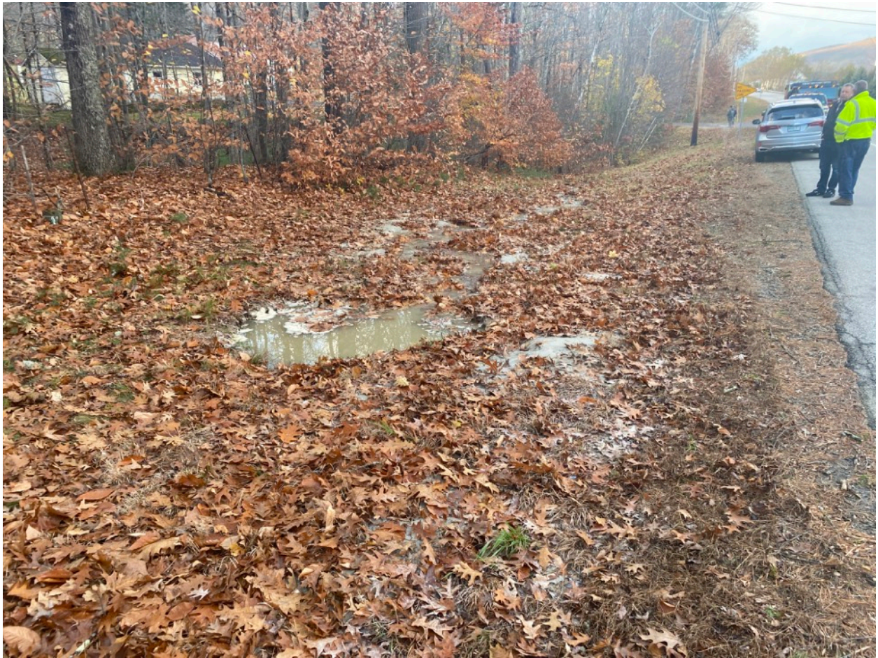
Fig. 1 - Clay-colored fluid collecting in and flowing out of an approximately 3 foot diameter hole and downhill in front of 183 Whittier Highway - 11/10/2023
