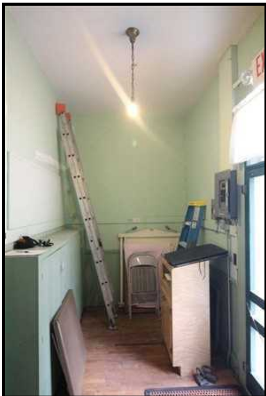
Image Interior Detail 006 – Interior at 1886 Schoolhouse Entry
