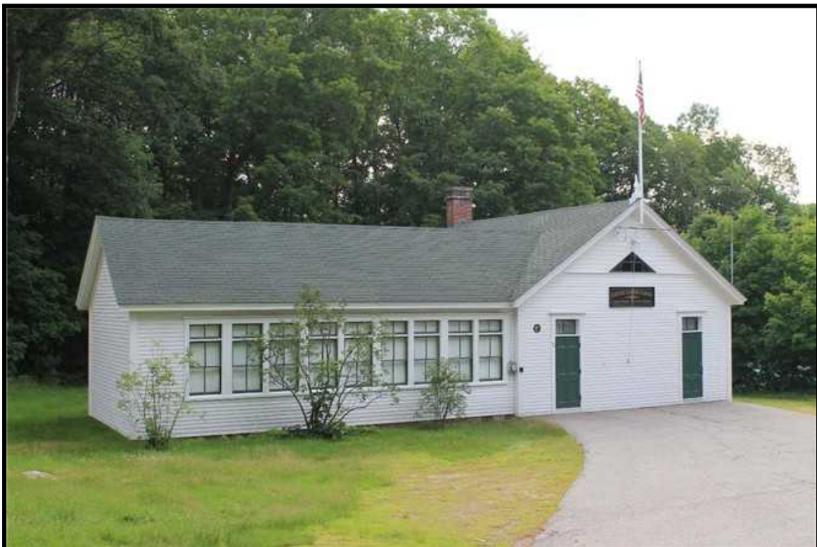
Image Exterior 004 – South West Elevation
