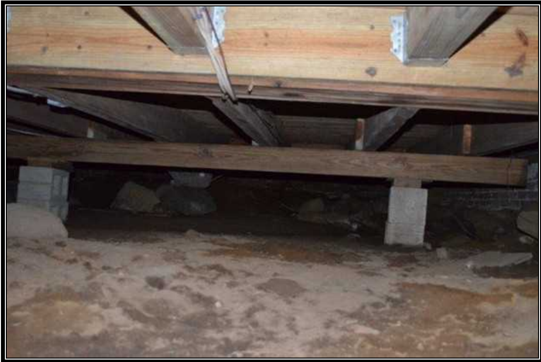
Photo 7: Repaired floor framing.
