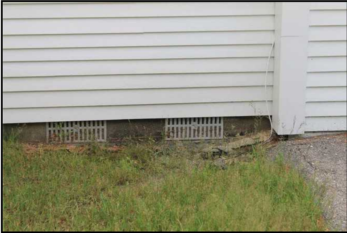
Image Exterior Detail 003 – Crawl Space Venting at 1902 / 29 Addition
