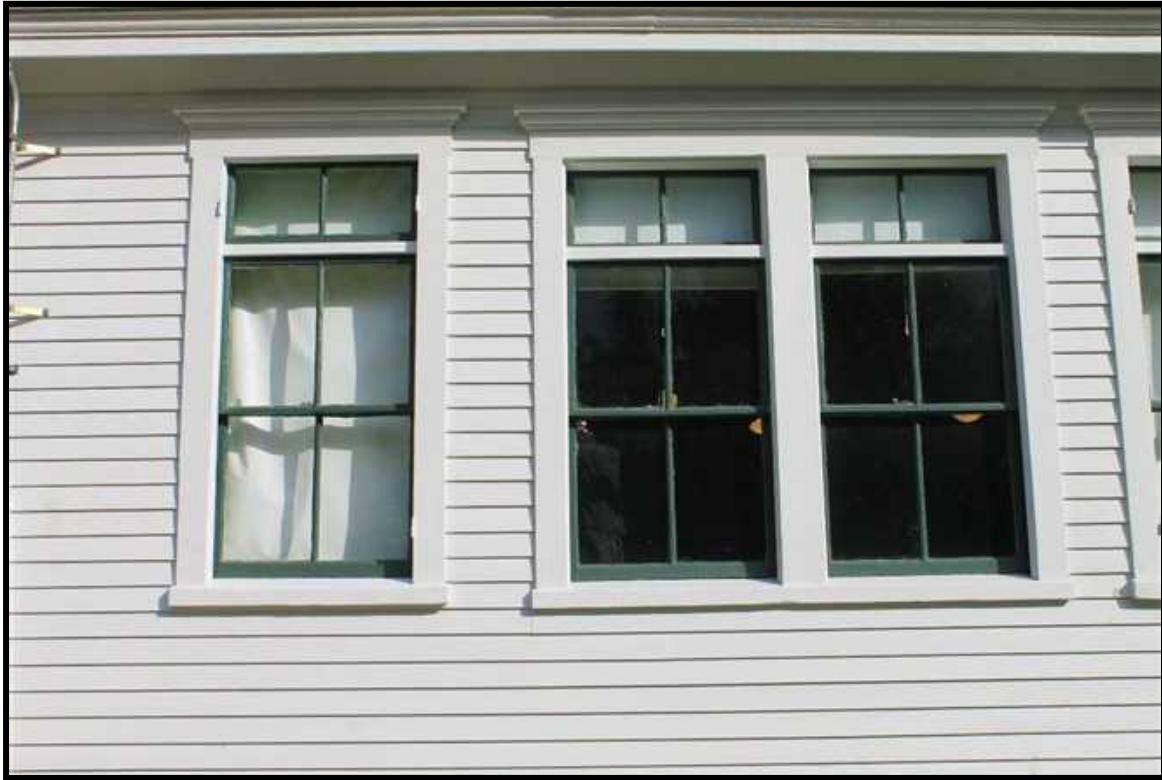
Image Exterior Detail 007 – Typical Windows at 1886 Schoolhouse
