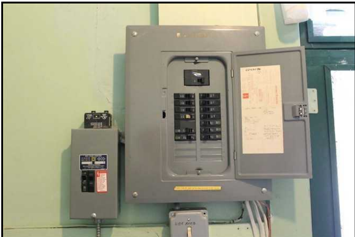
Image Interior Detail 010 – Existing Electrical Panel
