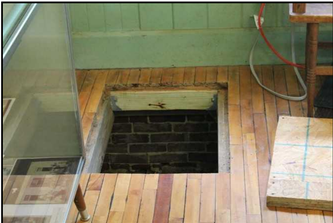
Image Interior Detail 004 – Crawl Space Access Hatch at 1886 Schoolhouse
