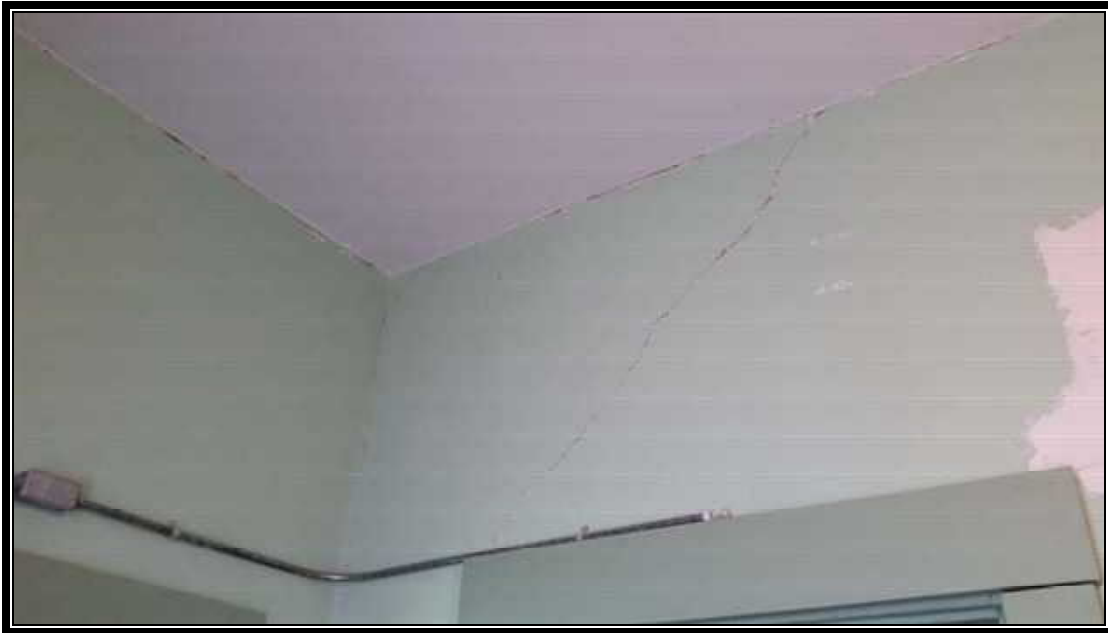
Photo 9: Cracks in the plaster on the inside of the front walls.
