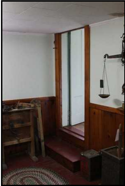
Image Interior Detail 005 – Floor Elevation Transition at Workshop Addition
