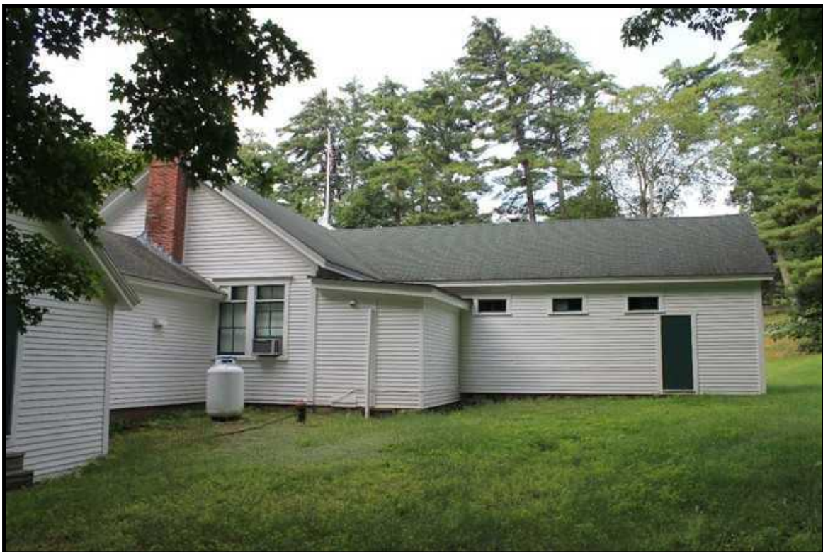
Image Exterior 006 – North East Elevation
