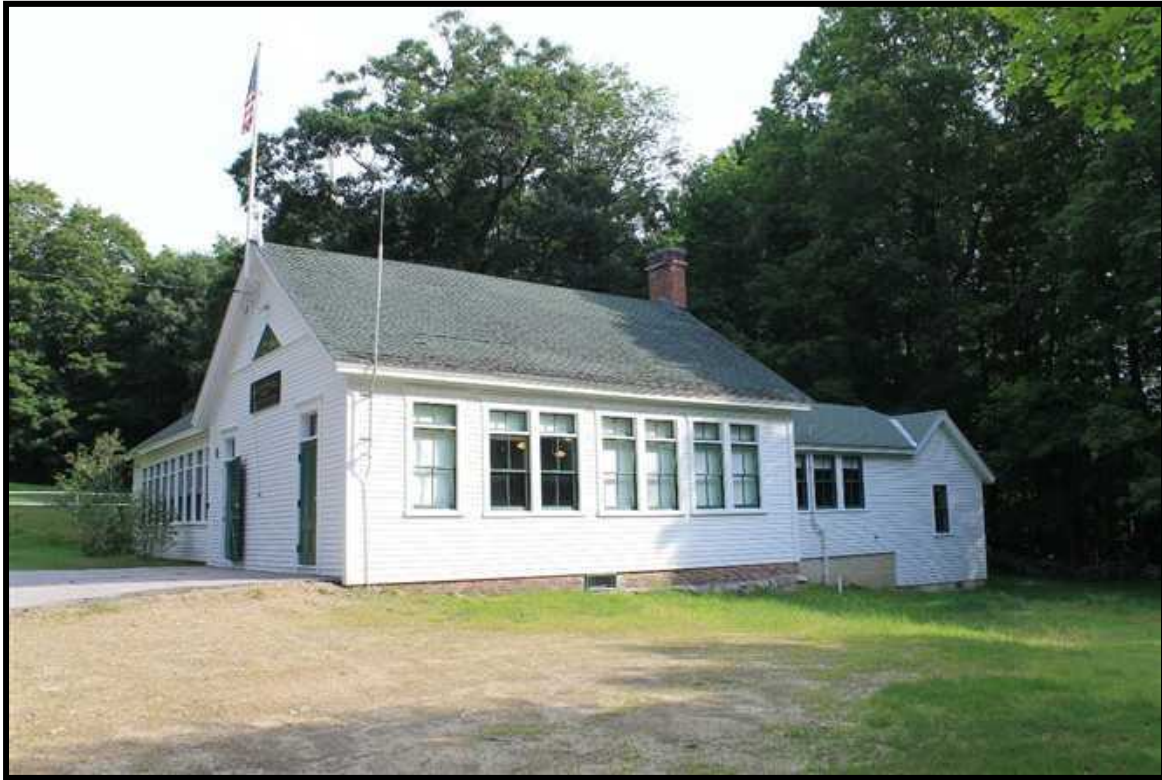
Image Exterior 009 – South East Elevation
