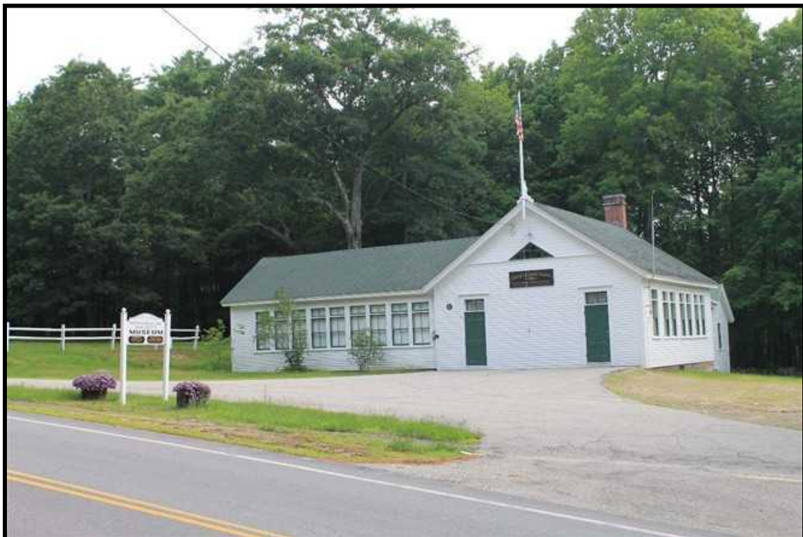
Image Exterior 002 – South West Elevation
