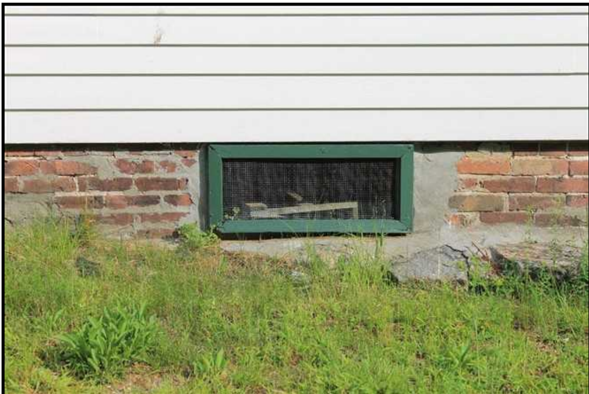
Image Exterior Detail 004 – Crawl Space Venting at 1886 Schoolhouse
