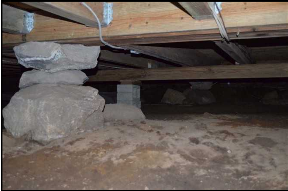
Image Interior Detail 013 - Crawl Space under 1886 Schoolhouse
