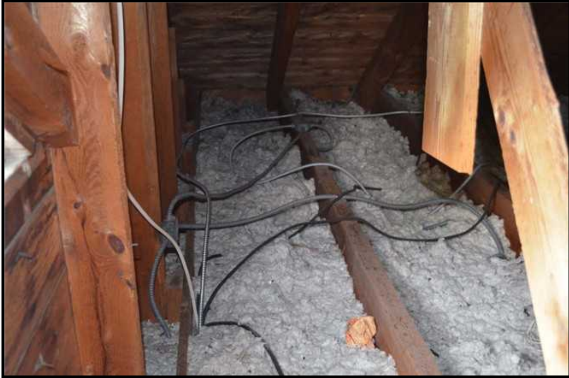
Image Interior Detail 015 - Attic above 1886 Schoolhouse
