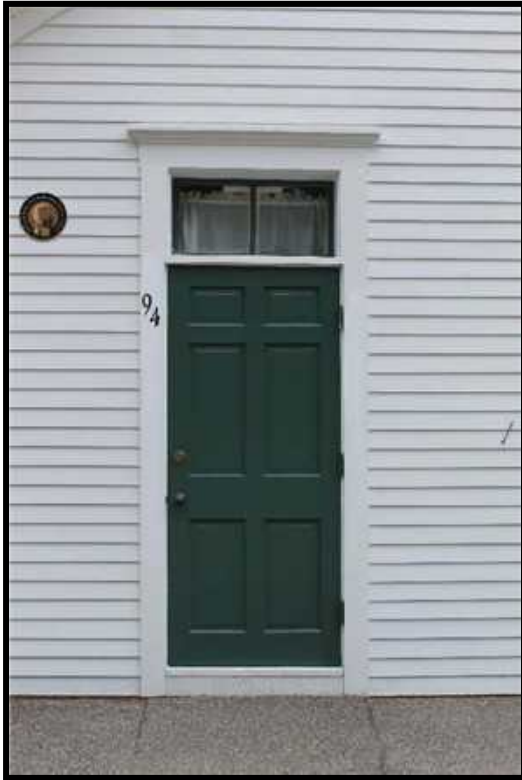
Image Exterior Detail 005 – Typical Door at 1886 Schoolhouse
