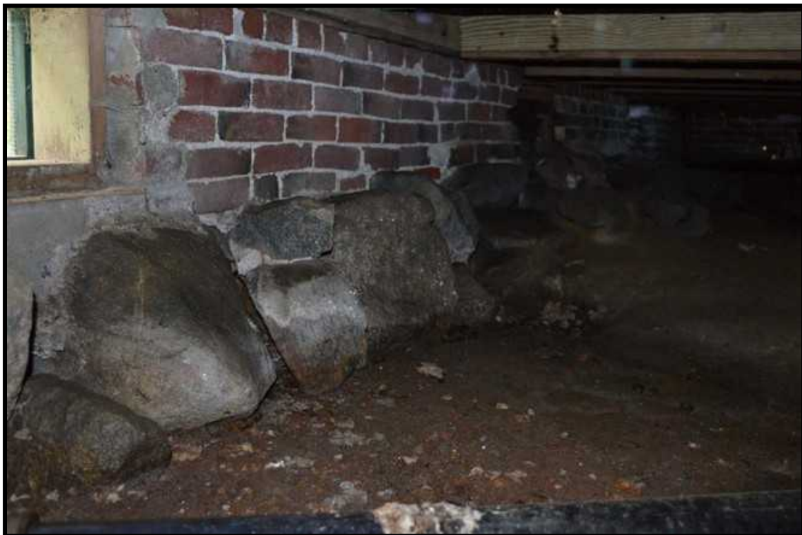
Image Interior Detail 012 – Crawl Space under 1886 Schoolhouse
