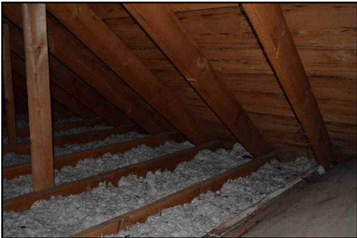
Image Interior Detail 014 – Attic above 1886 Schoolhouse
