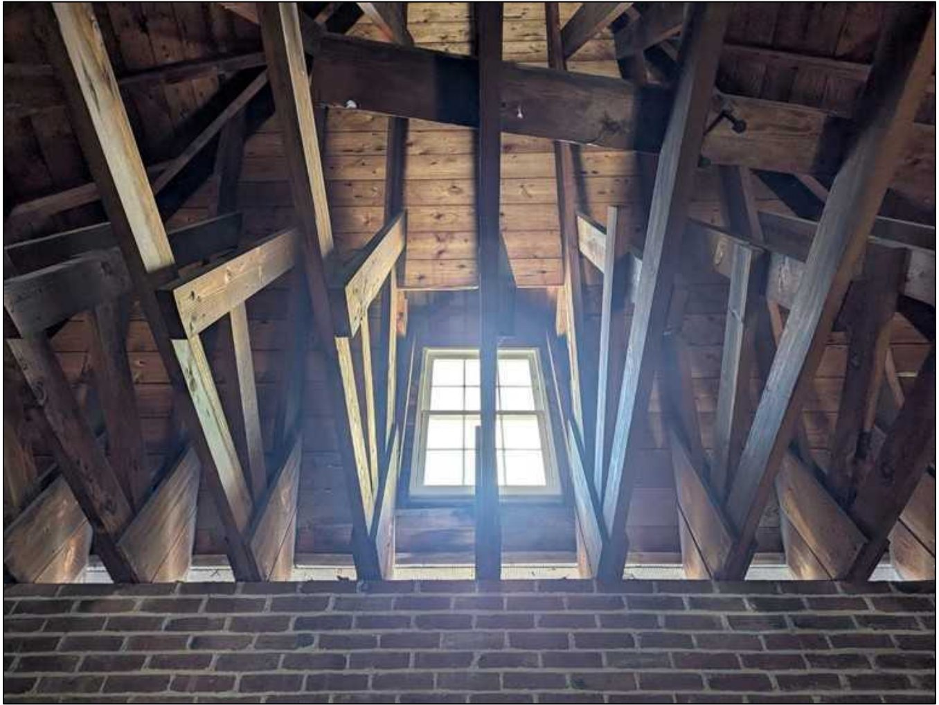
Photo 5: Canoe House roof truss system
